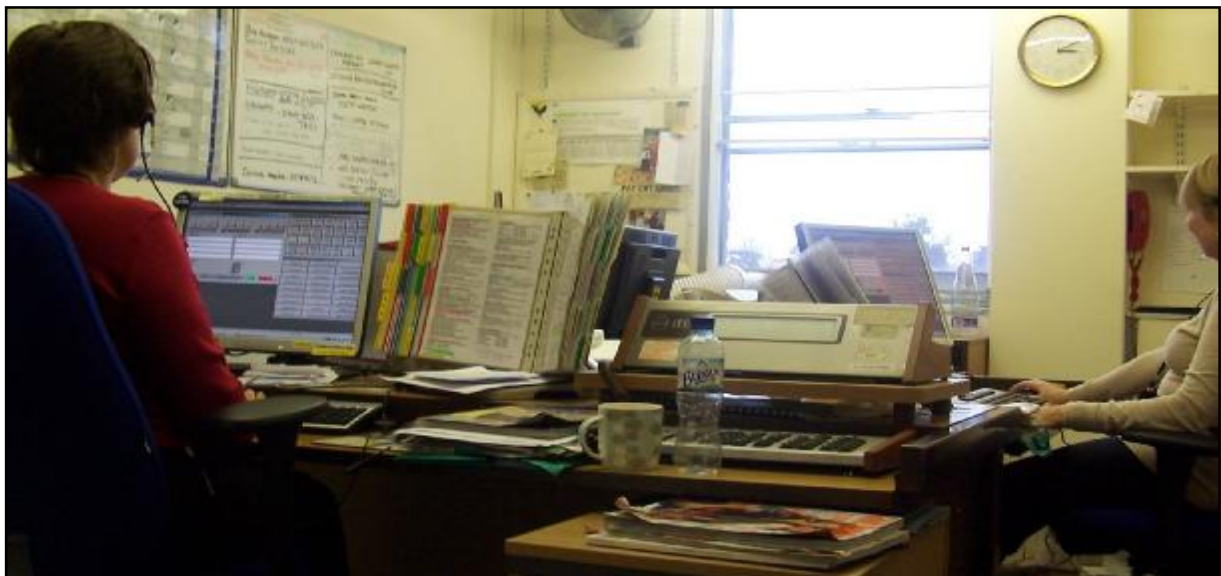
EFDC's switchboard is housed in a small room on the first floor of the Civic Offices
